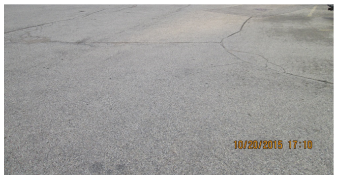
The asphalt parking lot is in poor to fair condition with some areas showing crocodile cracking. Asphalt repair, resurfacing and paint stripping will be required.
